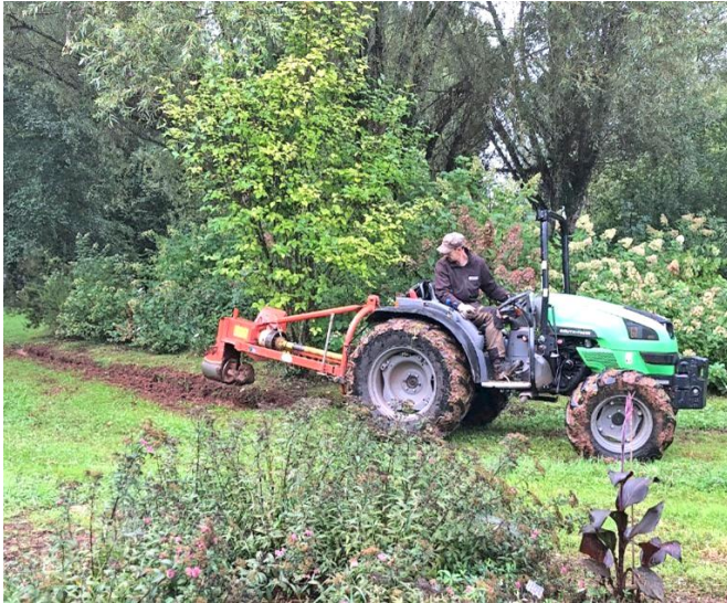
Fig 3. Digging ditches for drainage
